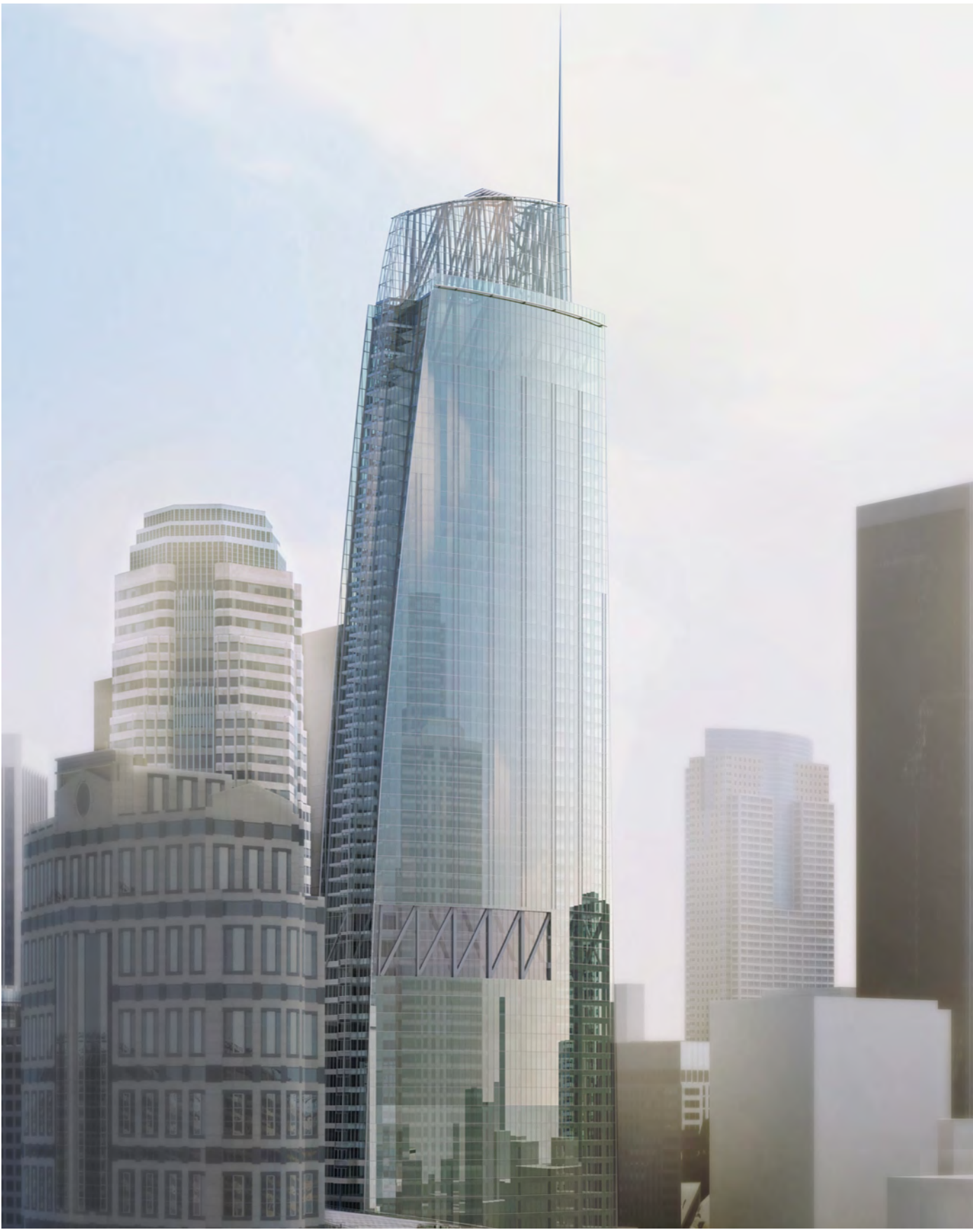
Wilshire Grand Center in Los Angeles, California. Currently under construction, foundation laid in 2014. Courtesy of the Internet.
